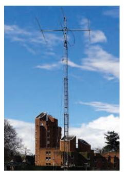
The 20m monobander + WARC dipole used for GR100MGY operations.
