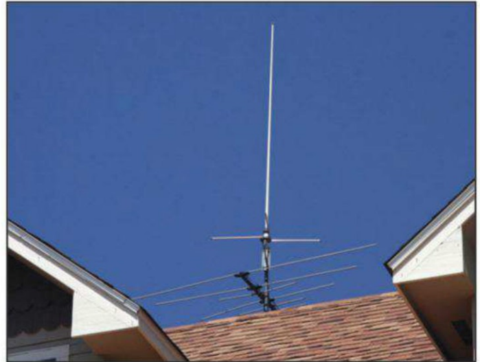
Photo 3. This dualband 2M/70 cm antenna is installed on top of the house, sharing the same mast as a TV antenna.
